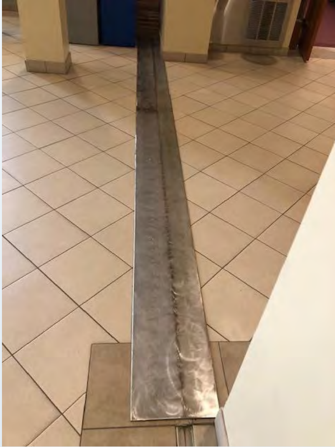
Stainless steel expansion joint cover installed in the gallery to protect the ceramic tiles
