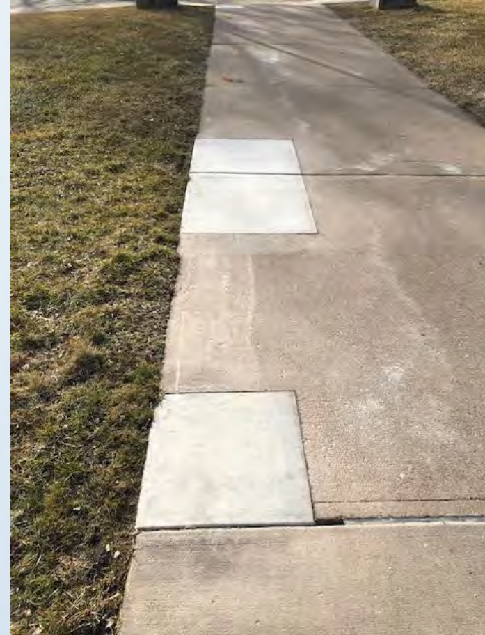
Sidewalk concrete repairs
