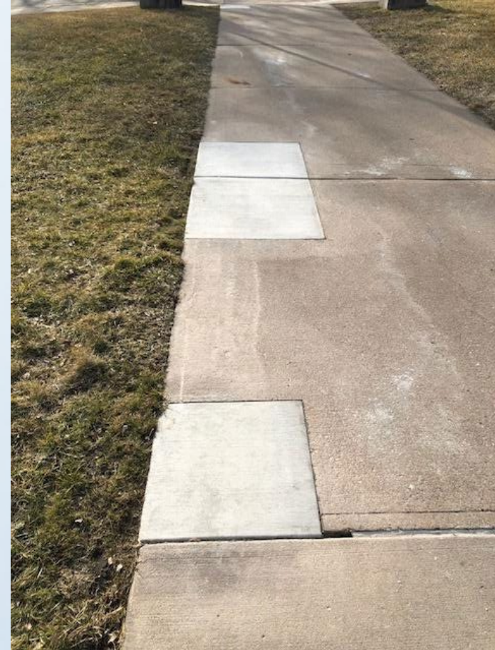
Sidewalk concrete repairs
