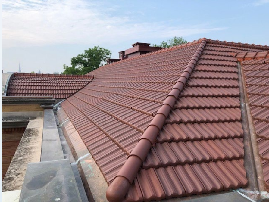
Original Roof replaced
