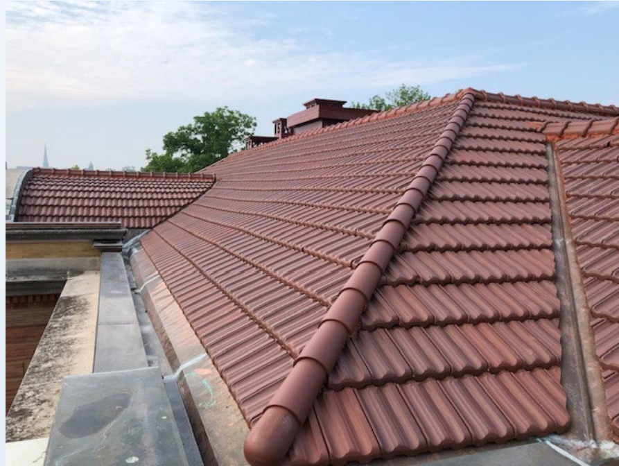
Original Roof replaced
