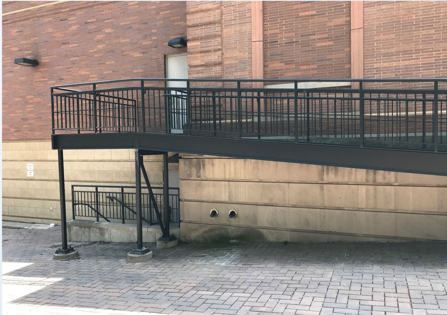
Repair and repaint catering ramp (under review now)
