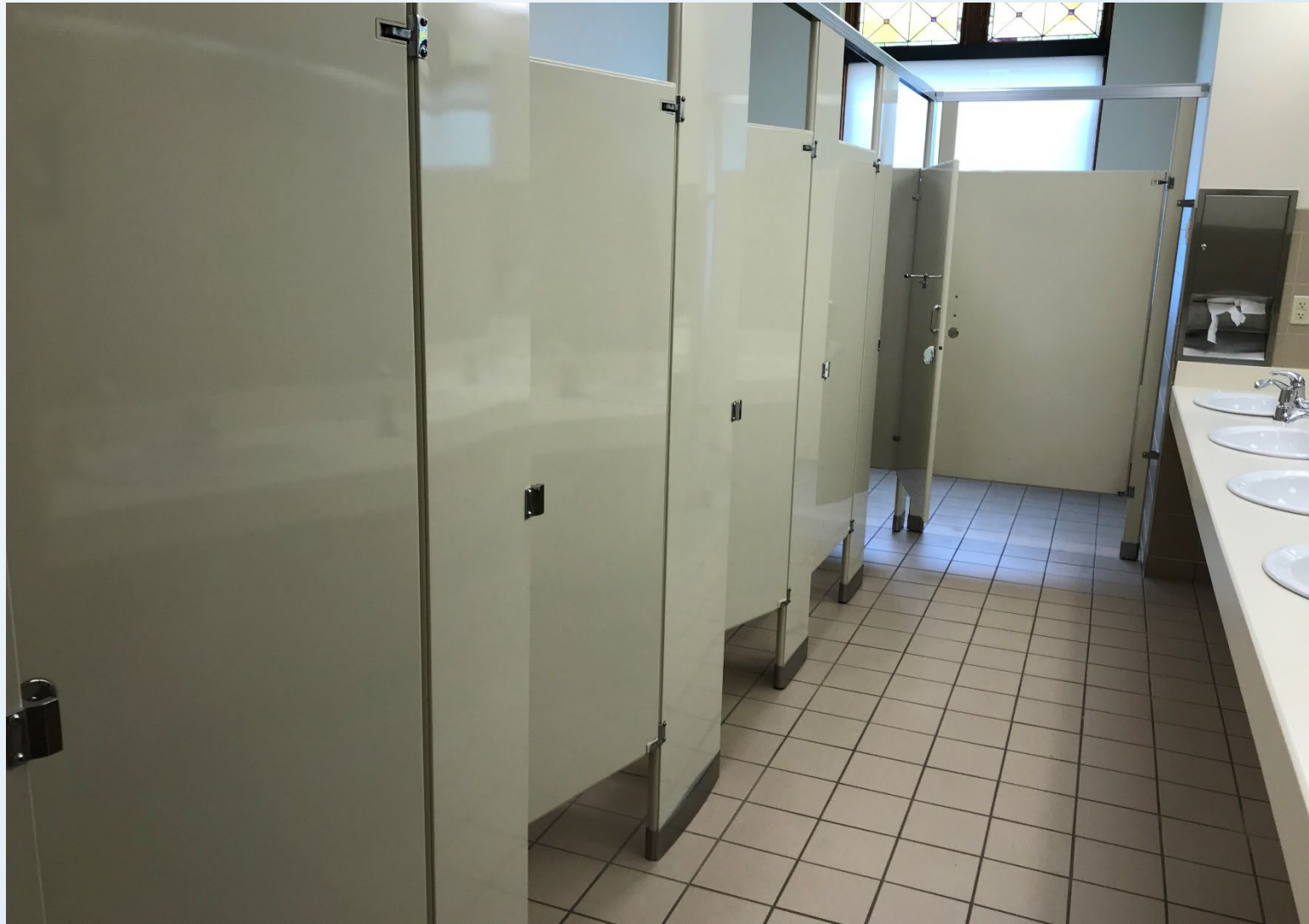
Restroom refresh with stall partition replacement
