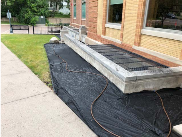
Halfway done; new landscape cloth is in place:
