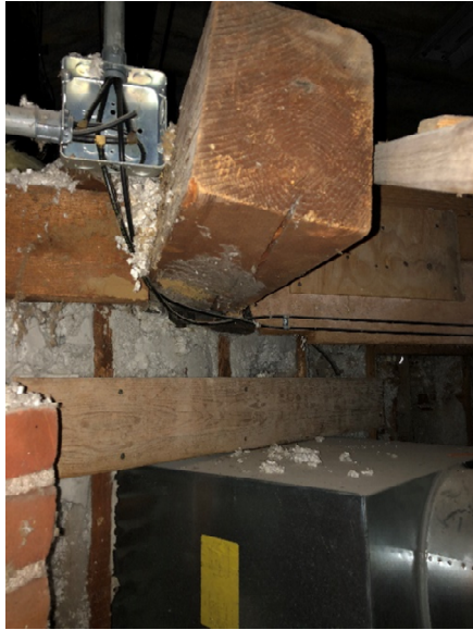
Photograph 4 Rolled Ceiling Beam
